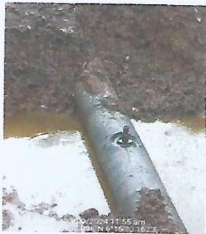
Pic1: Showing one (1no.) 2" nipple illegally installed on the pipeline
