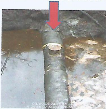
Pic1: Showing one (1no.) 2" nipple illegally installed on the pipeline
